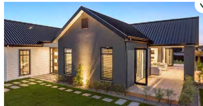
Soft lighting highlights the gabled elevation feature on this home.
