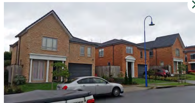
These homes do not have a strong street presence. Small openings, features aren't well considered, and neighbouring homes are too similar in appearance.
