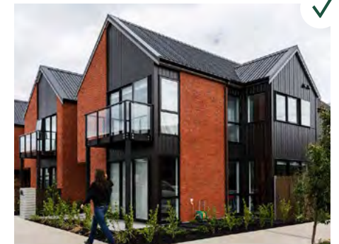
This two storey home has street presence by defining the street, and by having balanced streetscape elevations broken down with large openings
