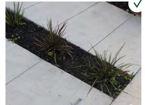
Decorative cuts and planting are encouraged for street appeal and driveway safety.
