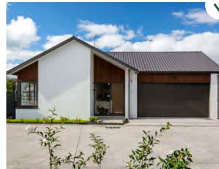
This home has a primary gabled form facing out to the street, and a secondary form (garage) attached.
