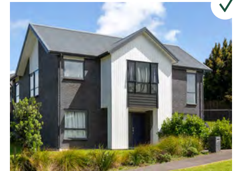
The upper floor of this home has the same footprint as the lower floor.
