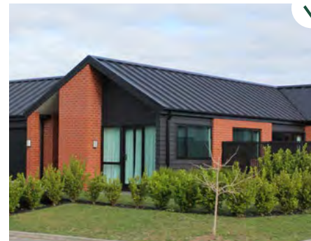
The down-pipe on the corner of this home does not stand out because it is of a material and colour that compliments the rest of the home.
