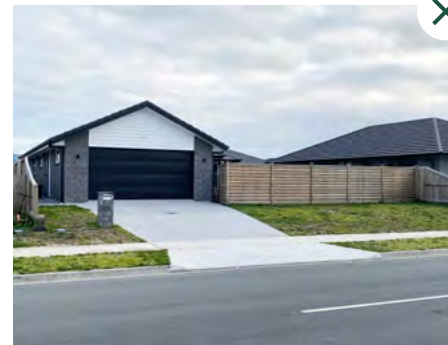
This home only has a garage fronting onto the street. This does not create an engaging street presence.
