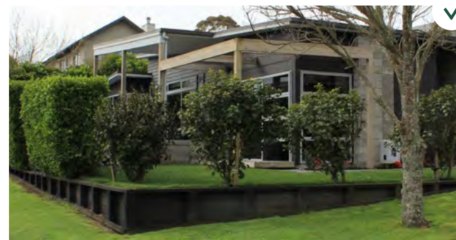
Retaining walls must be stained in a dark recessive colour to allow natural and other built features to stand out.
