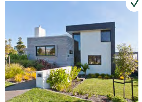
Letterbox incorporated into a blade wall beside the entrance path.
