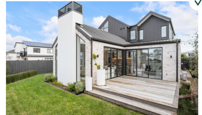
Decking is stepped down from the living room to be at a closer level to the natural ground level.
