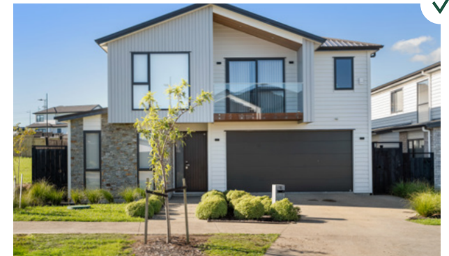
This home has a visually light glass balustrade with a top rail that allows people to lean on.
