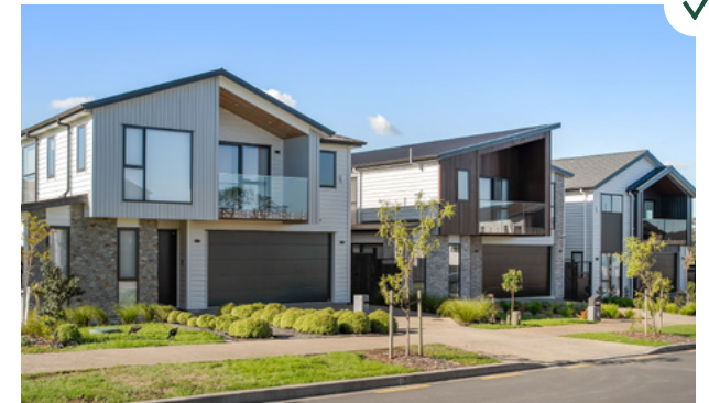
Variation in building form is encouraged in order to create an attractive neighbourhood character.
