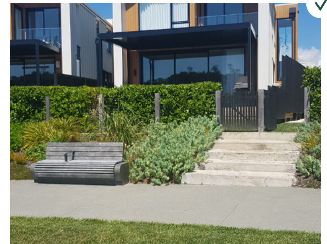
This illustrates an access from a reserve to the rear of the dwelling.
