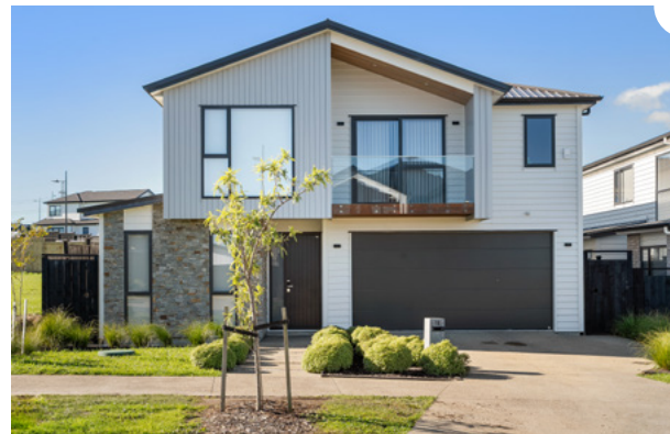
This home uses changes in material and recessed entry to create strong articulation and a defined street presence.
