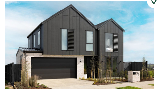
The down-pipe of this home does not stand out because it is of a material and colour that compliments the rest of the home.
