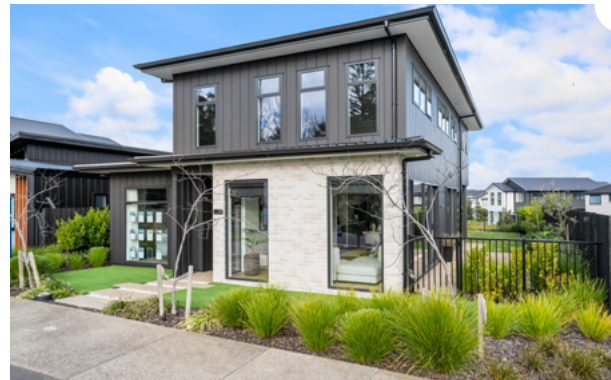
The habitable rooms of this house are facing North allowing for reasonable exposure to daylight.
